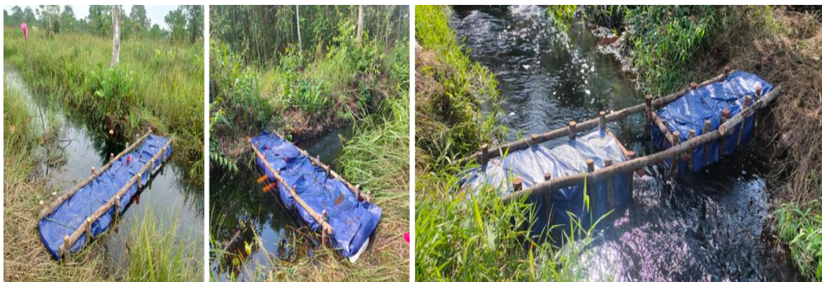
Constructed canal blocks at FC 99 & 100 (RMFR), Selangor
