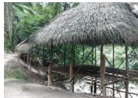
Construction of a mini chalet is well underway
