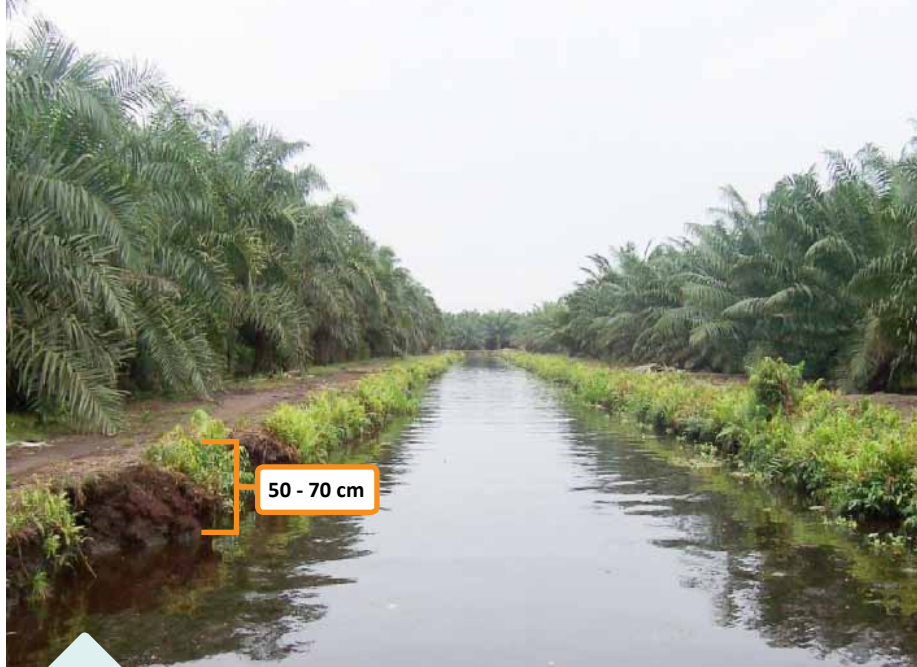
Figure 2.1: Water measured at collection drain needs to be in a range of 50 – 70 cm (Credit: Global Environment Centre, GEC)
