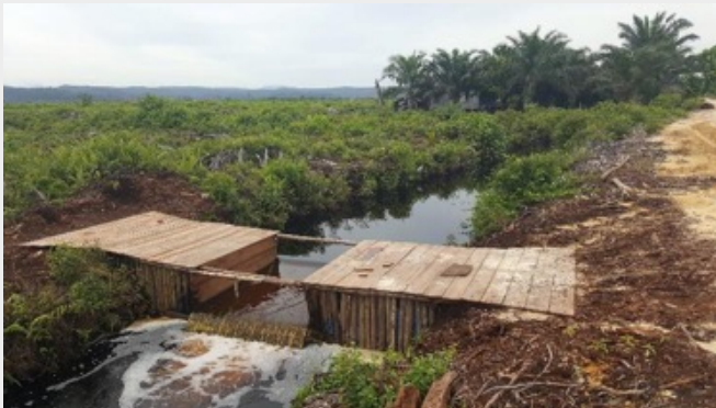
Gambar 2.4: Struktur pengendali air. (Sumber gambar: Ministry of Environment dan Forestry, Indonesia)
